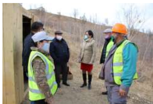
COVID-19 protocols being observed at the project site in Tunkhel village (photo taken by planetGOLD Mongolia)
