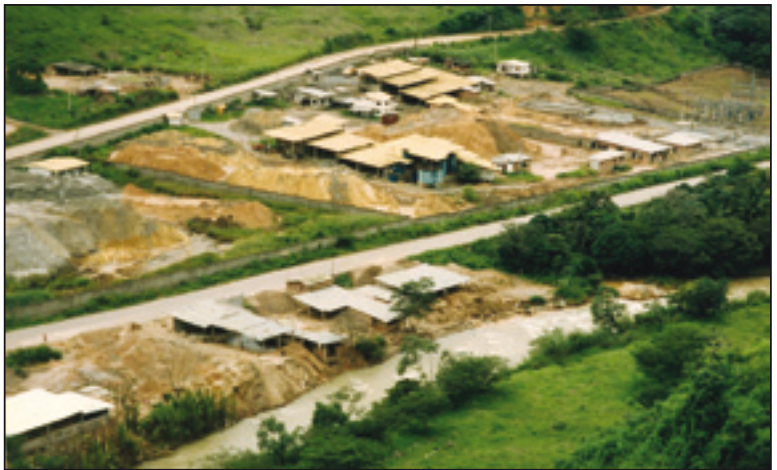
Figure 10: Mineral processing plants in the Rio Calera valley in Portovelo, Ecuador. (PMSC 1996)
